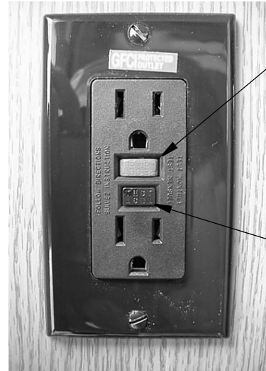
GFCI Outlet (Ground Fault Protector)
