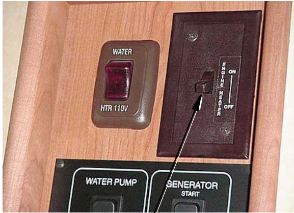
Diesel Engine Heater Switch (Typical)
