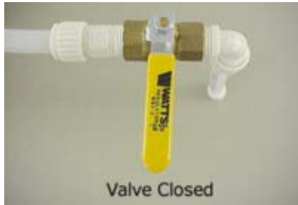
Water Tank Drain Valve (Typical) Under Rear Bed or Couch
