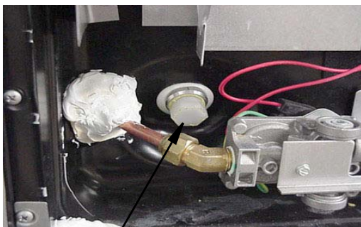
Water Heater Drain Plug Remove with socket.
