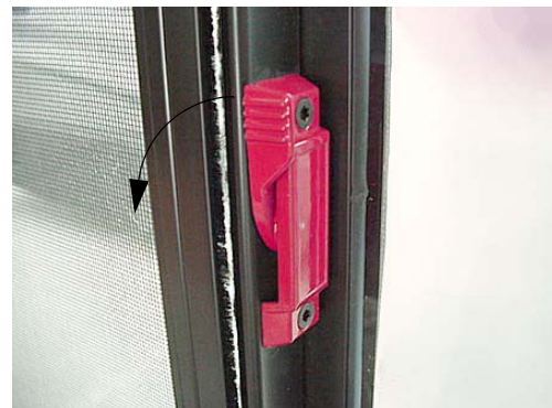
Pull latch outward to slide window open
