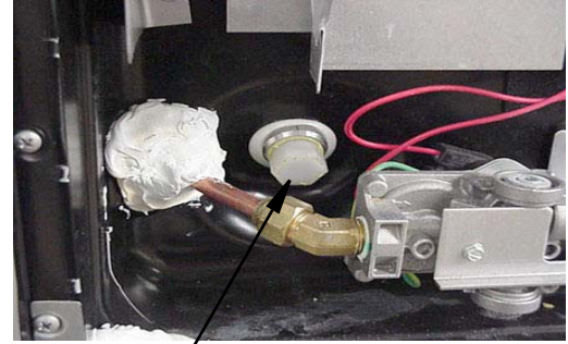
Water Heater Drain Plug Remove with socket.
