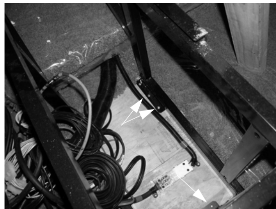
Steel Frame Screw Locations -Typical View
