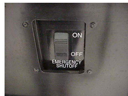
Main Tank Valve in Tank Fill Compartment
