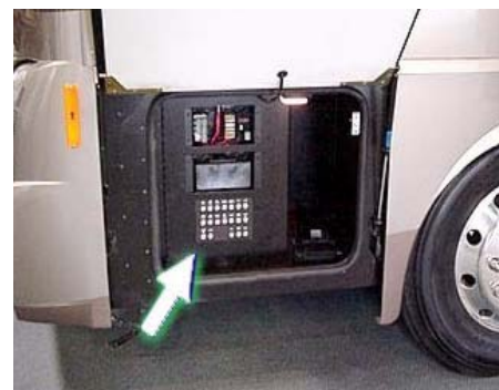
12V Electrical Compartment
