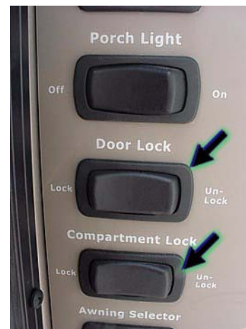
Power Door Locks on entry switch panel
