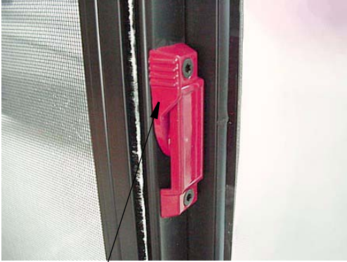
Pull latch outward to slide window open
