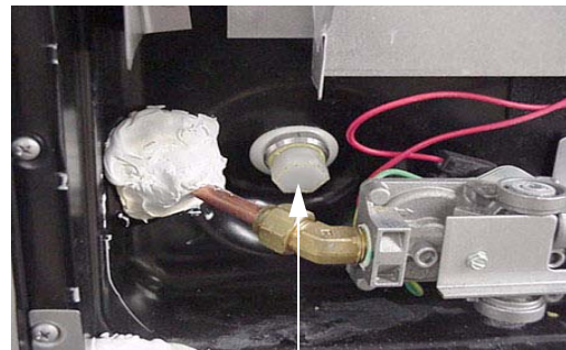
Water Heater Drain Plug (Remove with socket)
