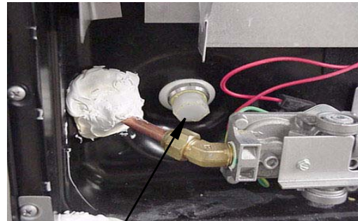
Water Heater Drain Plug Remove with socket
