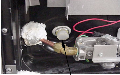
Water Heater Drain Plug Remove with socket.
