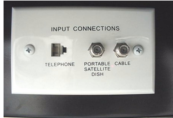
Exterior Connection for Satellite Dish and Cable TV (In Water Center or Shoreline Compartment)
