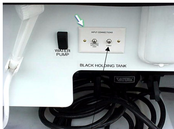
Cable TV Hook-Up in Utility Compartment
