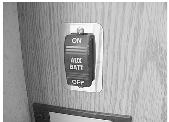
Aux. Batt. Switch (Near entrance door)
