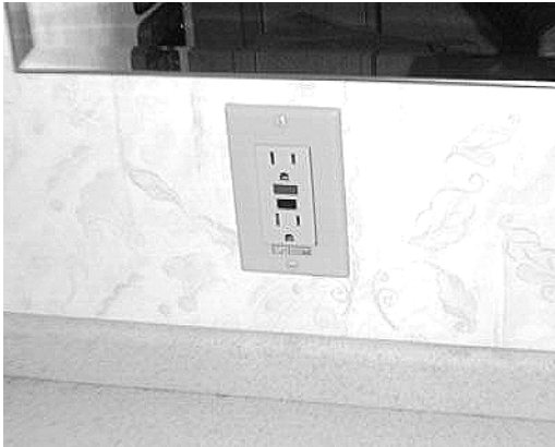
Ground Fault Circuit Interrupter (GFCI)
