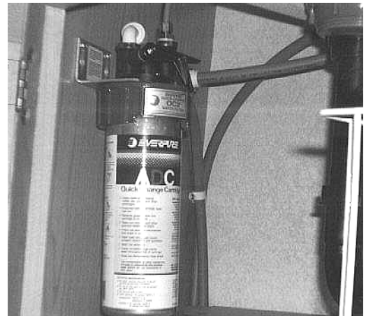
Water Filter Assembly - Below Galley Sink
