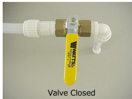
Water Tank Drain Closed
