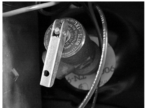
Lift straight out to open P-T valve
