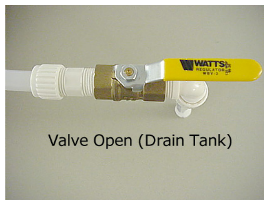
Water Tank Drain Open
