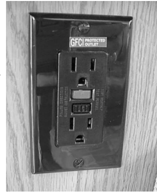
GFCI Outlet (Ground Fault Protector)
