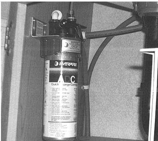
Water Filter Assembly - Below Galley Sink
