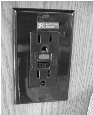
GFCI Outlet (Ground Fault Protector)
