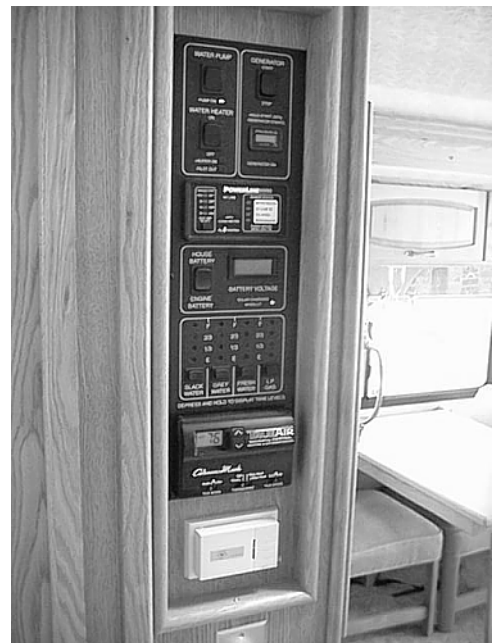
One Place Monitor Panel
