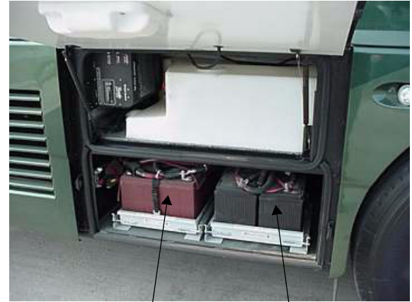
Chassis Batteries House Batteries
