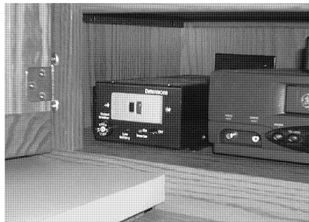
DC-AC Voltage Inverter in Video Center
