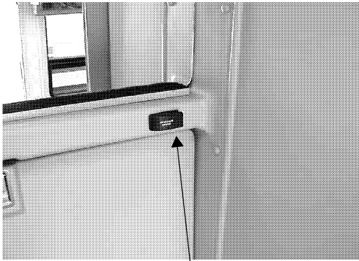
Shower Drain Pump Switch
