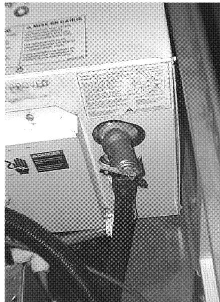
Pressure-Temperature Relief (P-T) Valve
