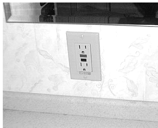
Ground Fault Circuit Interrupter (GFCI) below bathroom mirror
