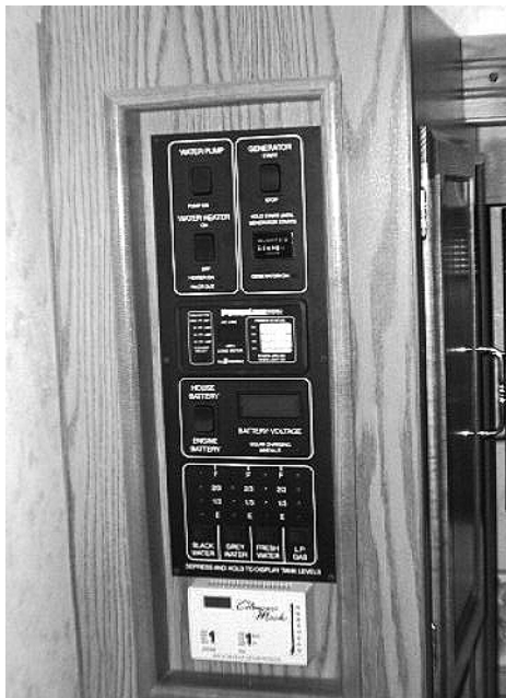
Monitor Panel - Model 38KD In Hallway Across From Refrigerator
