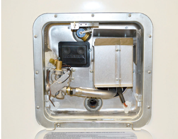
Water Heater Exterior Service Access
