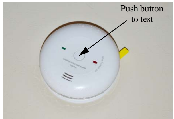
Carbon Monoxide Alarm
