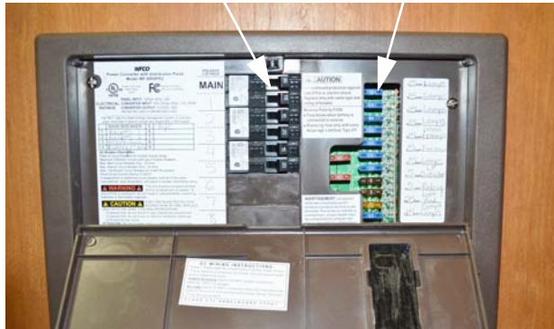
Power Center (Converter) -Typical View
