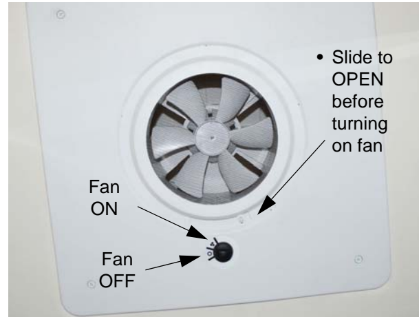
Power Roof Ventilator
