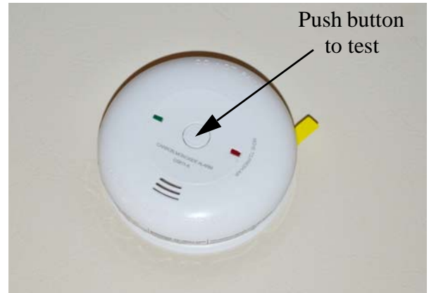
Carbon Monoxide Alarm
