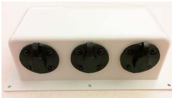
3-Port Solar Cap (Located on the roof)
