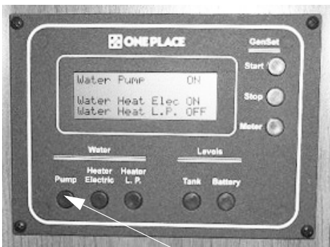
Water Pump Switch
