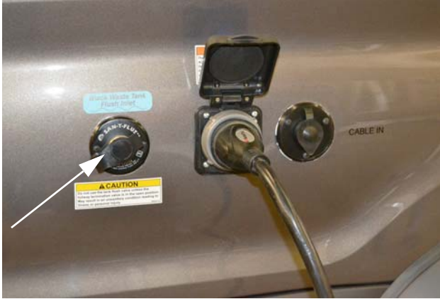
Black Waste Tank Flush Inlet (Located on driver sidewall)
