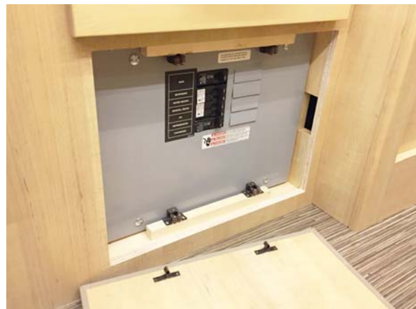
120-Volt Circuit Breakers -Typical View
