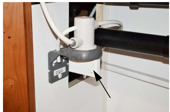
Diverter Plug (installed in filter socket)
