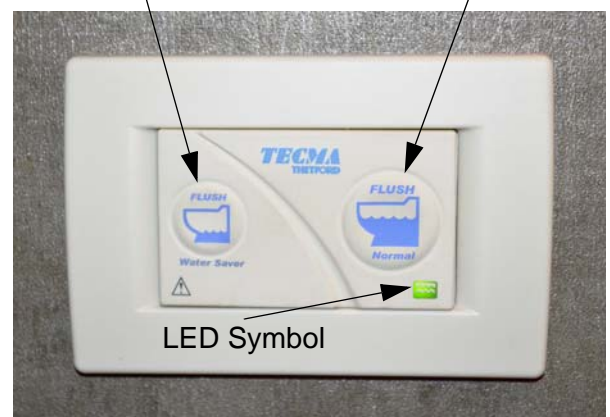
Wall Switch/Controller (Located on wall near toilet)
