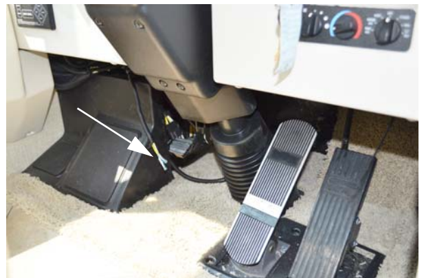
CB Power Wires -Typical View
