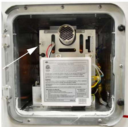
Water Heater Power Switch (Located inside water heater door) -If Equipped
