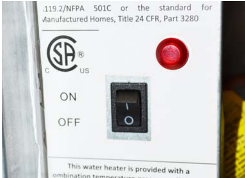
Water Heater (Tankless) Power Switch -If Equipped
