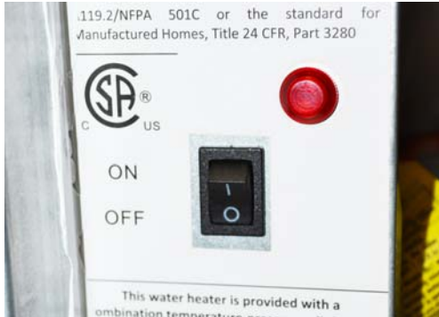
Water Heater (Tankless) Power Switch -If Equipped
