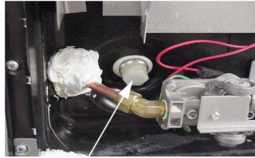
Water Heater Drain Plug (Remove with socket)
