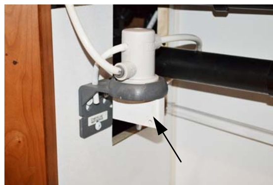
Diverter Plug (installed in filter socket)
