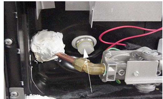
Water Heater Drain Plug (Remove with socket)
