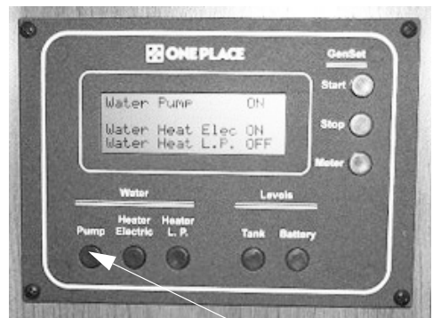
Water Pump Switch
