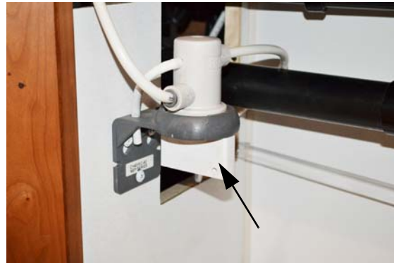
Diverter Plug (installed in filter socket)
