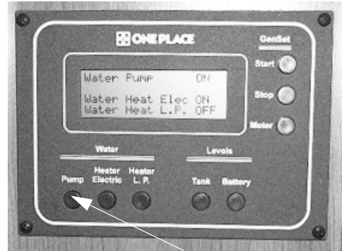
Water Pump Switch
