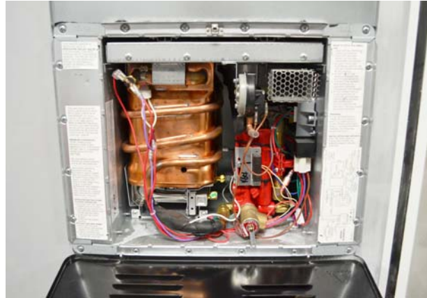
Water Heater Exterior Service Access -Typical View
