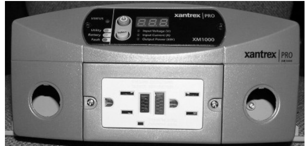
Inverter Unit (Located inside an exterior compartment) -Typical View
