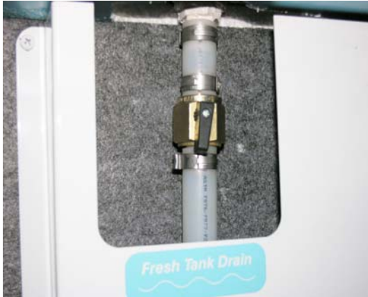
Water Tank Drain Valve -Typical Installation
