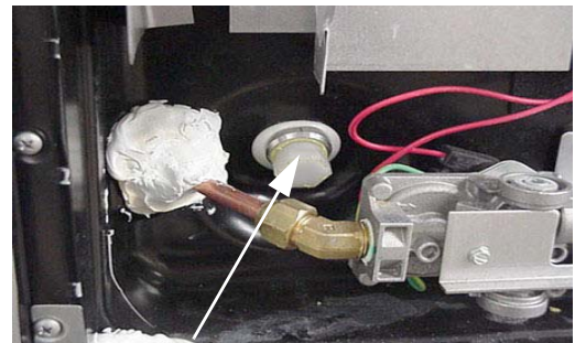
Water Heater Drain Plug (Remove with socket)
