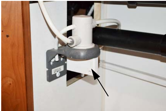
Diverter Plug (installed in filter socket)
