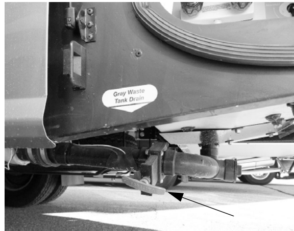
Gray Waste Tank Drain Valve (Located beneath rear driver side of coach) -Typical View
