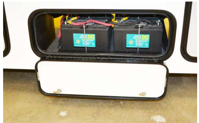
House Batteries (located behind a driver side exterior door) *Model 31C shown
