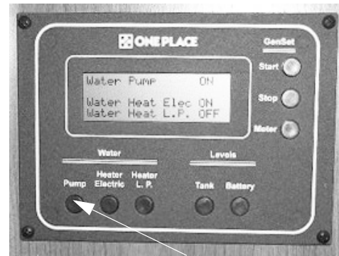
Water Pump Switch
