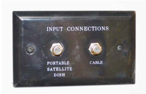
Cable TV and Portable Satellite Connections (Located in the utility or shoreline compartment depending on model.)
