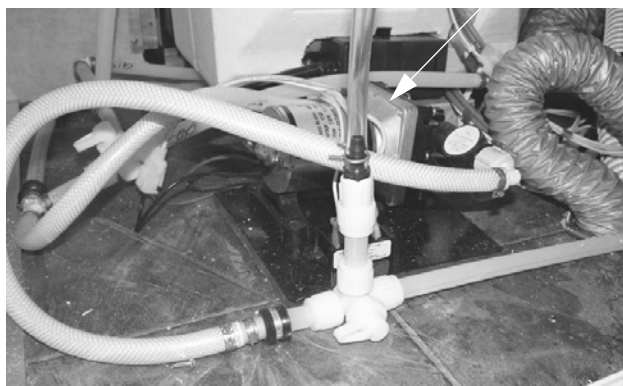
Water Pump (Located in backwall compartment. Remove side panel to access) -Model 24V shown
