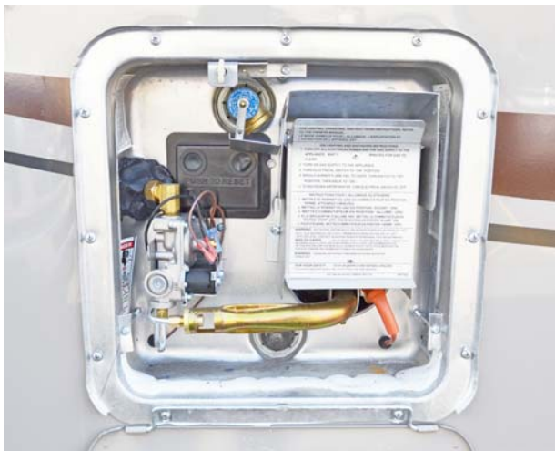
Water Heater Exterior Service Access
