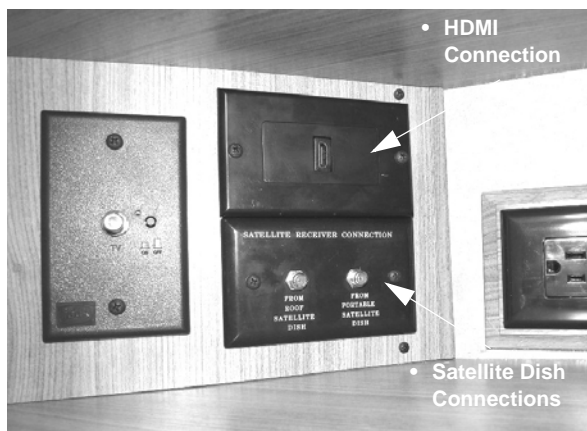
Interior Satellite Dish and HDMI Connections (Located near entertainment center cabinet) -Typical installation shown
