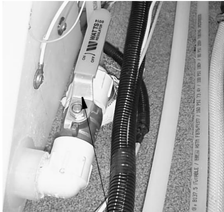
Water Tank Drain Valve (Typical)
