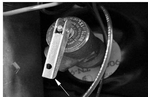
Pressure-Temperature Relief Valve
