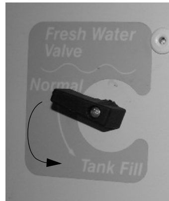
Fresh Water Valve (Located in water service center)
