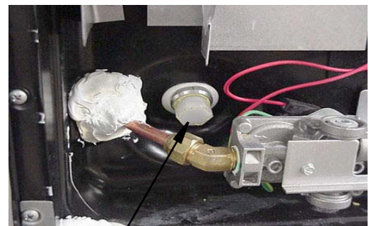
Water Heater Drain Plug (Remove with socket)
