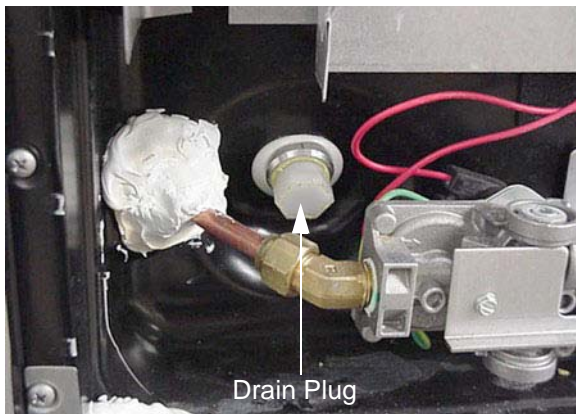
Water Heater Service Access -Typical View
