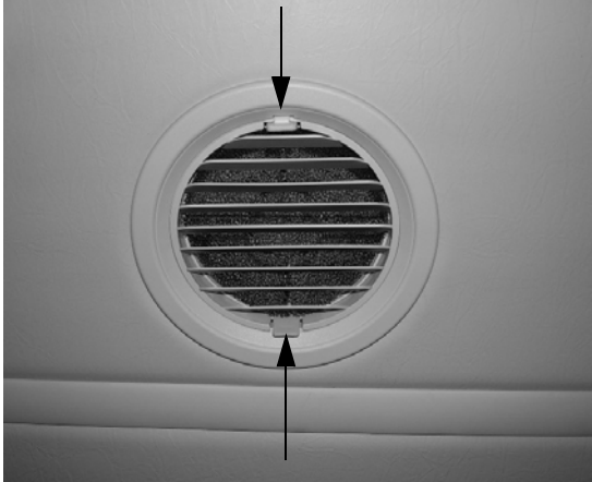
Return Air Vent (Press tabs inward to remove air vent)
