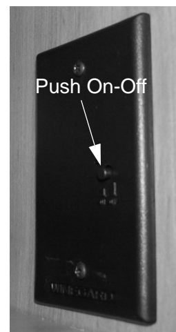
TV Signal Amplifier Switch (Located near entertainment center cabinet) -Typical View
