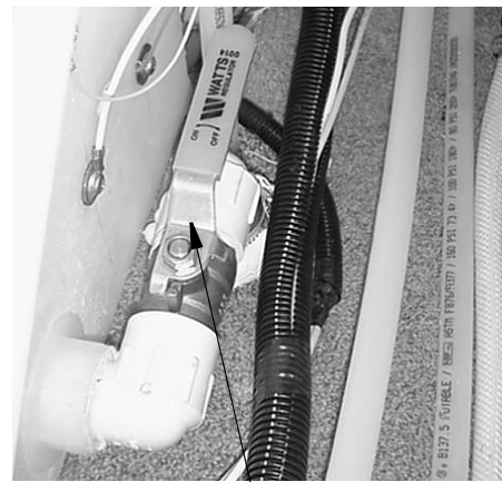
Water Tank Drain Valve -Typical Installation
