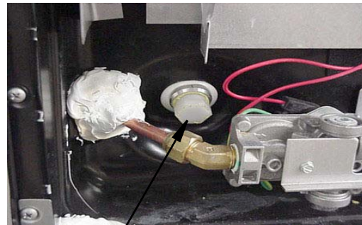
Water Heater Drain Plug (Remove with socket)
