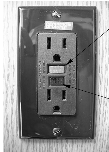
GFCI Outlet (Ground Fault Protector)
