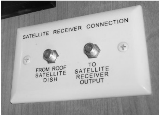
Interior Connection for Satellite Dishes (Located on wall or in cabinet near TV) -Typical View
