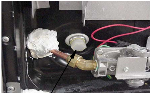
Water Heater Drain Plug (Remove with socket)
