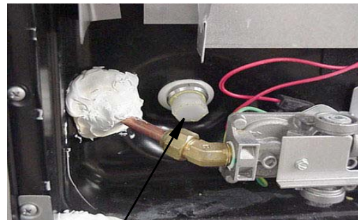
Water Heater Drain Plug (Remove with socket)
