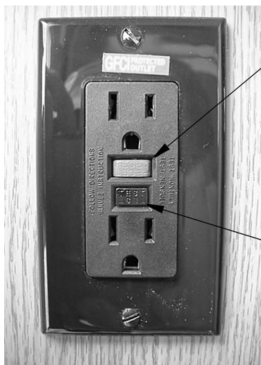
GFCI Outlet (Ground Fault Protector)
