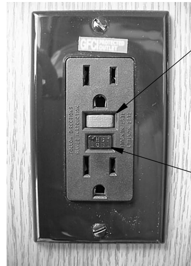
GFCI Outlet (Ground Fault Protector)
