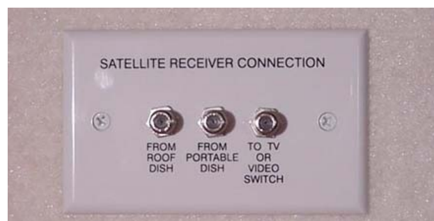
Interior Connection for Satellite Dishes (in cabinet near TV*)
