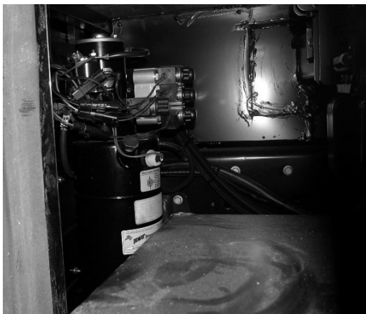
Hydraulic Pump (Behind driver's side cab) - Typical View
