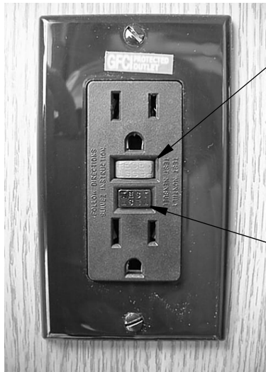
GFCI Outlet (Ground Fault Protector)
