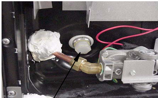
Water Heater Drain Plug Remove with socket.
