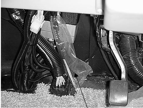
CB Power Wires (in plastic sheath)
