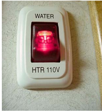
Electric Water Heater Switch (Typical)
