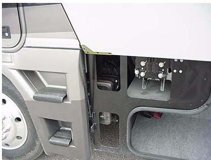
Hydraulic Pump Access - open storage compartment door behind driver's side front tire.
