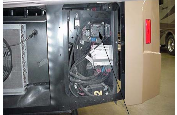
Towing Package fuses are on fuse block
