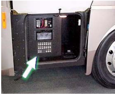
12V Electrical Compartment
