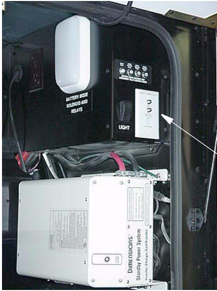
Exterior Input Connections for Satellite Dish, Cable TV and Phone in Water Center or Shoreline Compartment
