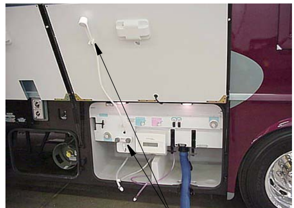
Exterior Wash Station/Shower
