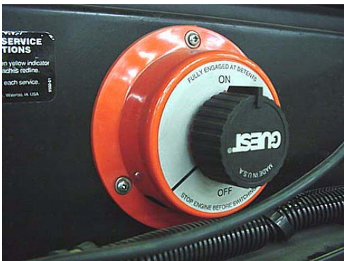
Chassis Battery Cutoff Switch inside rear engine access grille
