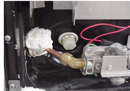
Also open the Pressure-Temperature relief valve at the top right portion of the tank to prevent air locking in the tank while draining.
