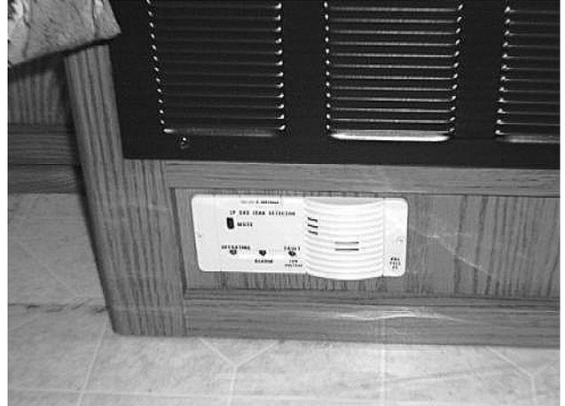
LP Gas Leak Detector
